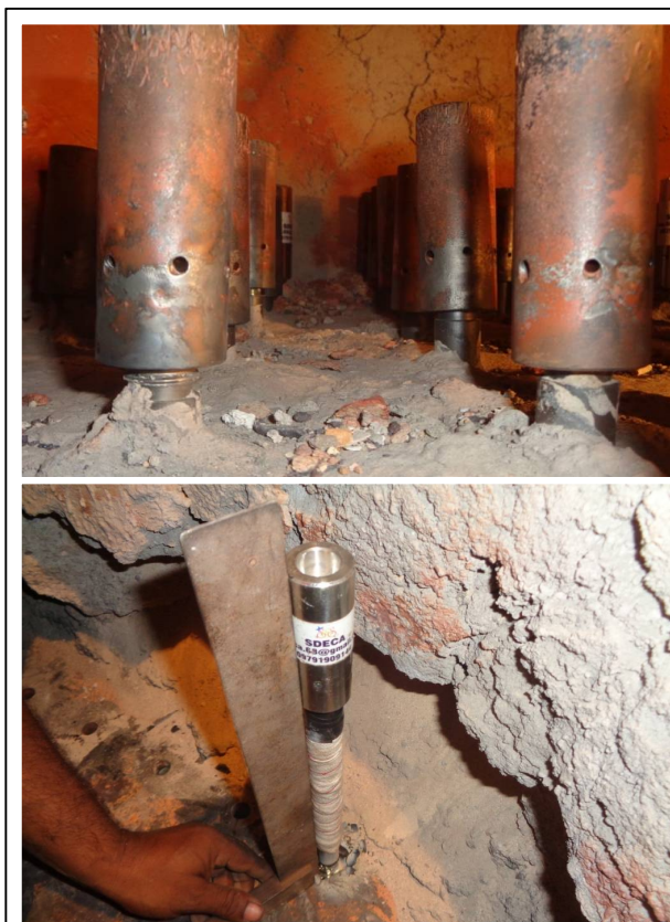
Photo 3 & 4 : Misfit nozzles ( earlier) and New nozzle ( being fitted).
